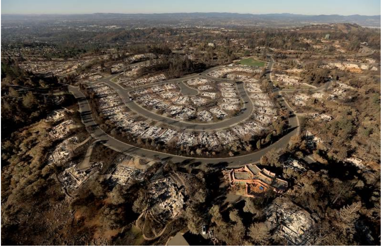
Fountaingrove, Santa Rosa, following the Tubbs Fire of October 2017.
