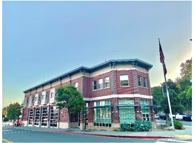
Station 1 333 Johnson Street, Sausalito
