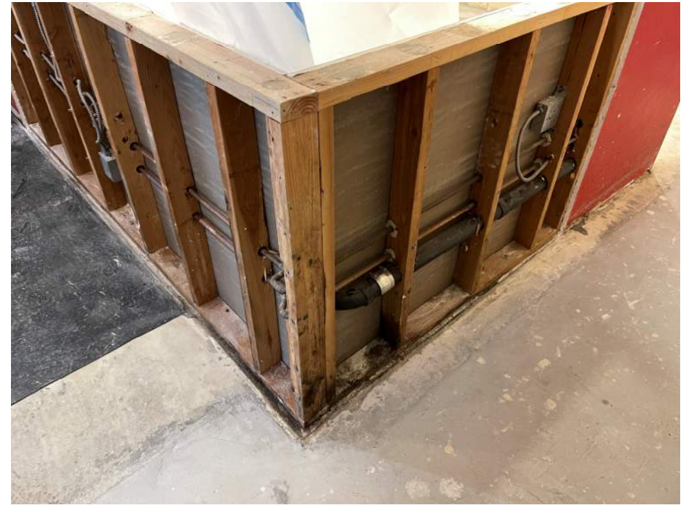
PHOTO 7: STUDS AT KITCHEN WALLS
