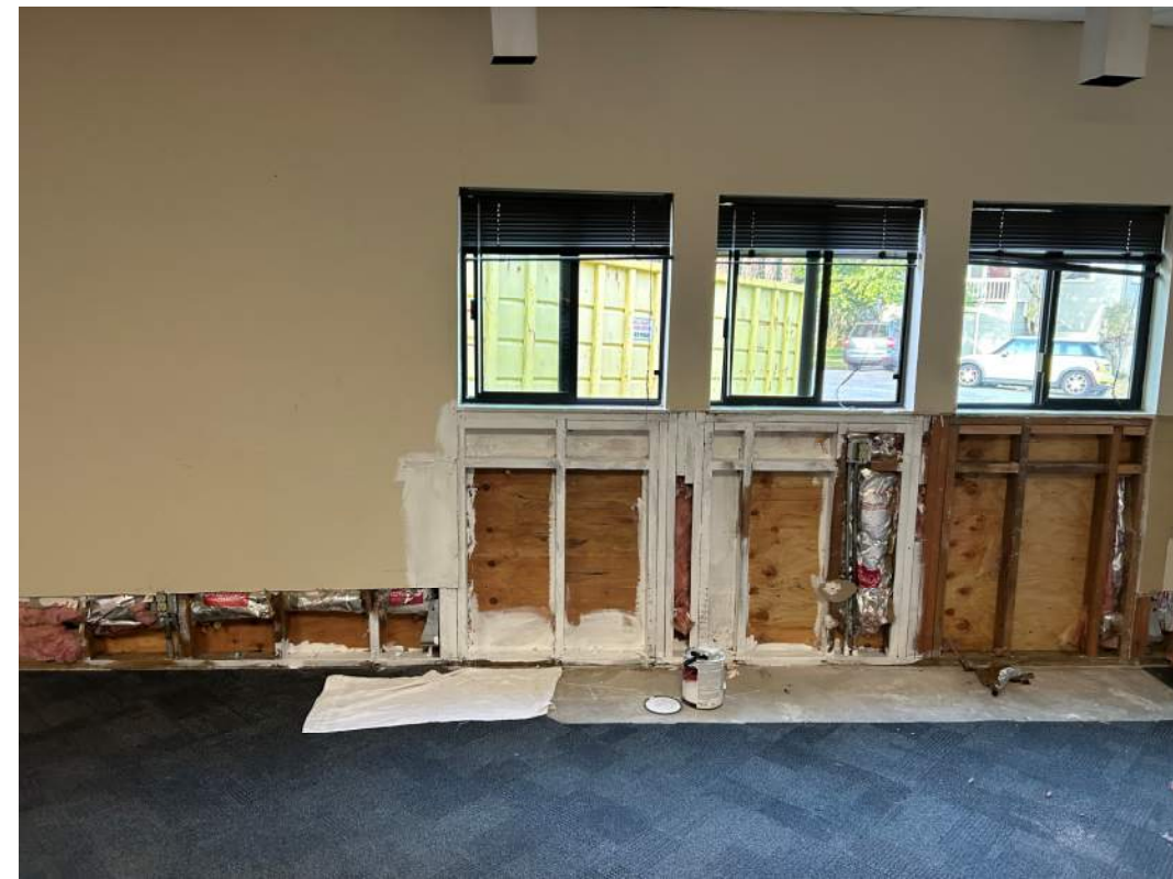
PHOTO 3: MOLD KILL PRIMER BEING APPLIED TO WALL
