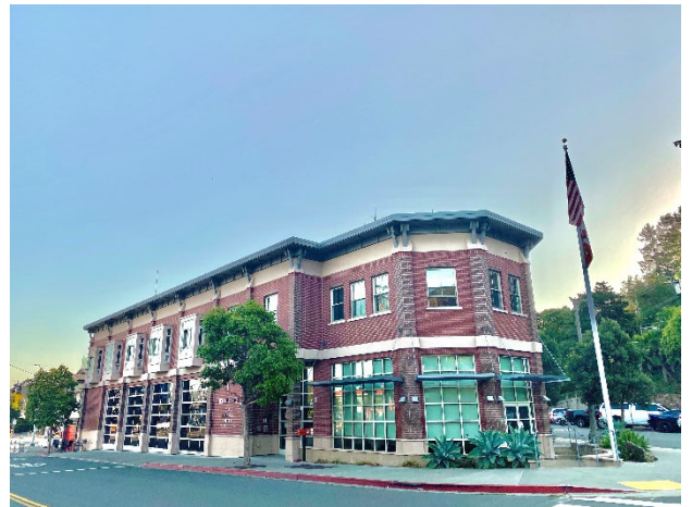
Station 1 333 Johnson Street, Sausalito
