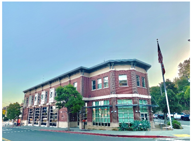
Station 1 333 Johnson Street, Sausalito
